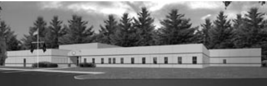
Consigli Construction has completed work on the Maine Army National Guard Readiness Center (above) with SMRT Architects...photo by SMRT
