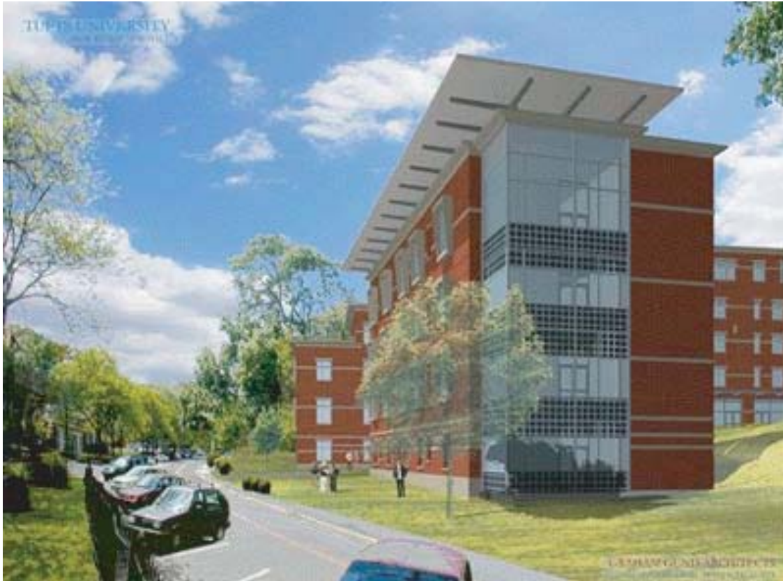
Tufts Solar Residence Hall Tufts University Medford, MA (LEED Silver Rating Anticipated)
