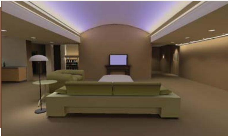
(Figure 6) Great Room Color-changing LED system is concealed in cove along each side of great room to uplight vaulted ceiling, and provide mood and circadian benefits; blue light has been found to be effective in activating the circadian system.
